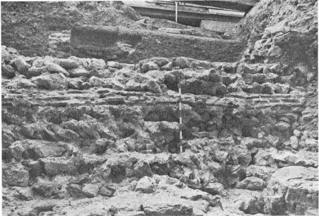
Fig. 8: View looking south. Longitudinal section through the Roman Wall showing details of the construction. (Photo: John Bailey)
