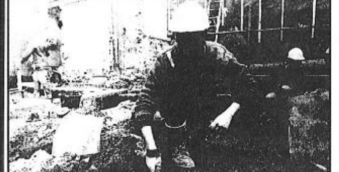
Scraping away layers of history in Leadenhall Street. (205424)
