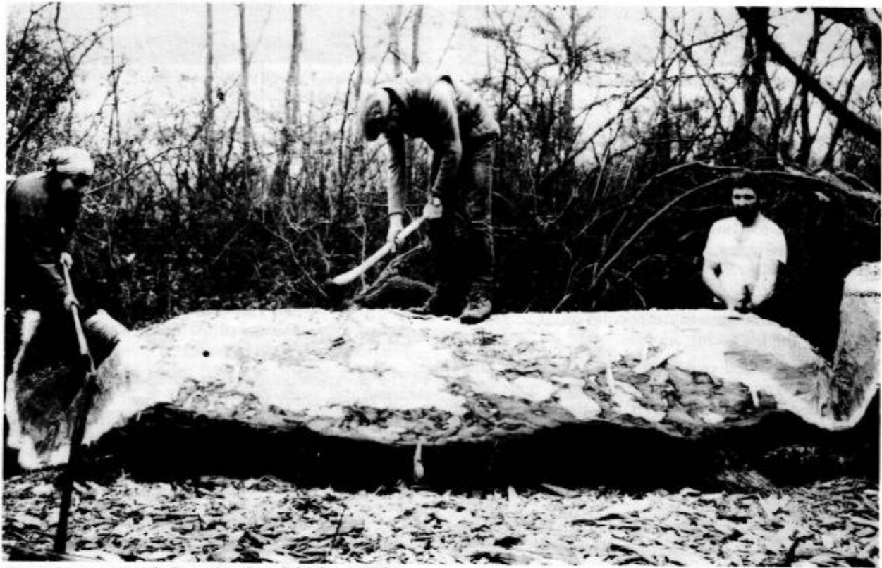
Fig. 3: Cross-cutting the log to length and shaping outside. (Photo: M.A.S.)
