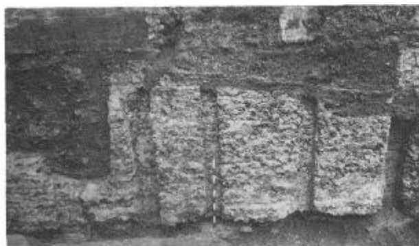
Fig. 6: Building A; looking south on new flint wall in south-east corner. One metre scale sits in one of five vertical slots rising from the horizontal slot at the base of the wall, possibly representing ghosts of timber shuttering.
