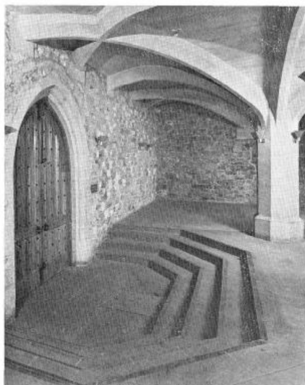
Fig. 5: Truncated vaulting at the east end of the west crypt. Both the vaulting and the floor have been restored, but the end of the vaulting had survived in the wall (left) which separated the two crypts. (Photo: T. Hurst)
