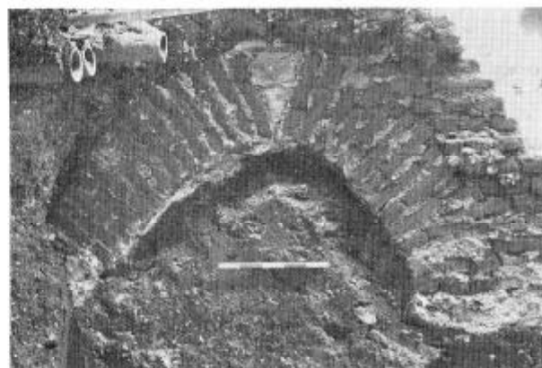
Fig. 8: The arched brick wall constructed up against the internal face of the City wall.
