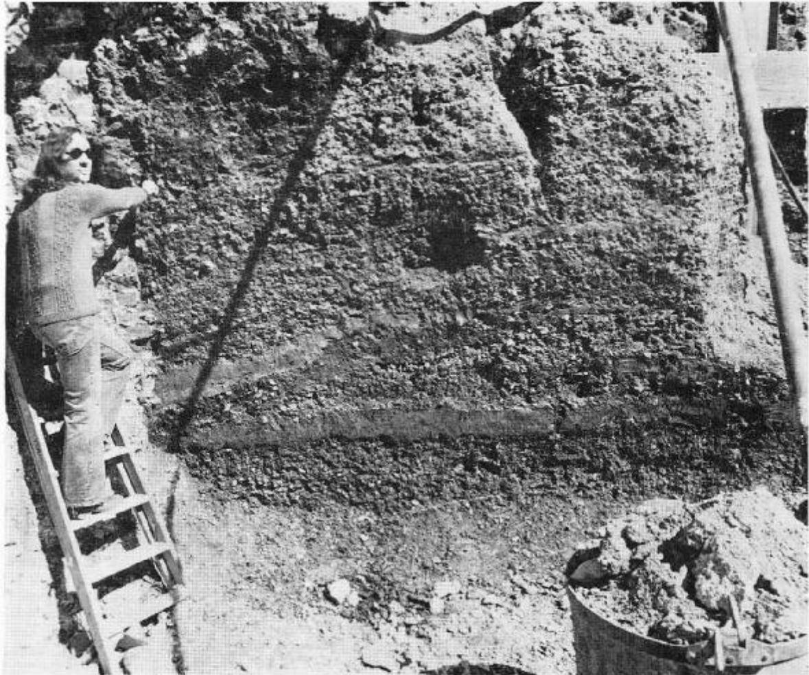
Fig. 1. The section of the Roman road north of Montague Chambers where the resurfacing produced a gravel thickness of 1.5 metres. (Photo: John Earp)
